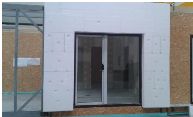
Obr. 12: OSB desky a polystyrenová izolace [5]
